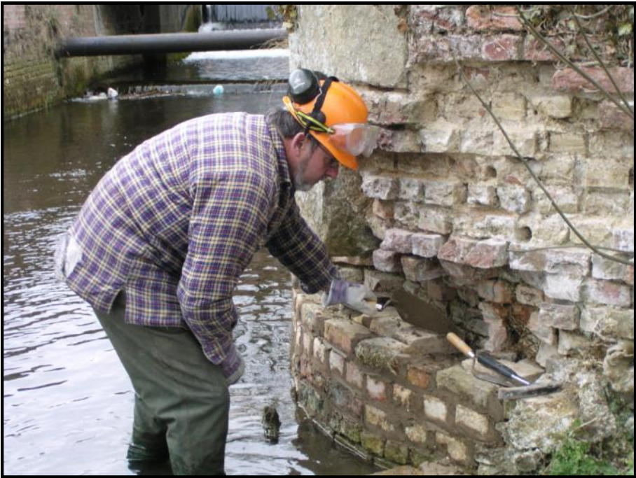
Dave Carnell. Repairing the wing walls at Cogglesford.
