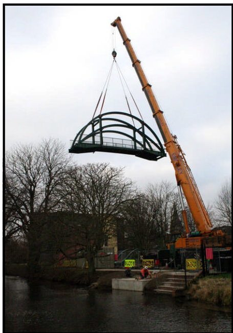
The bridge being lifted over the trees
