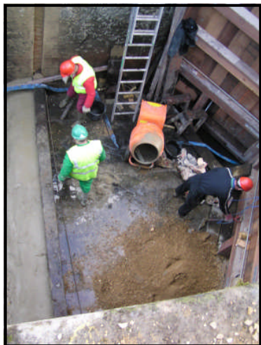
Trust members concreting stop board base
