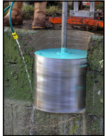
Cutting the lock ladder grooves
