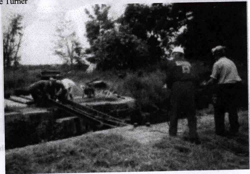
Constructing the barrow bridge at Haverholme. Photo courtesy of BITM.
