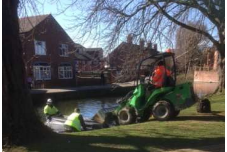
Sleford Town Council staff and contractors working on backfilling the coir rolls along the banks at Eastgate Green April 2018
